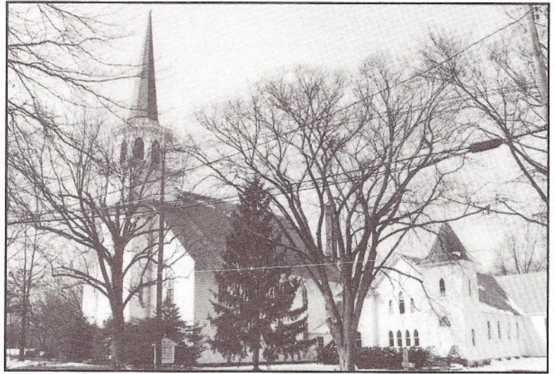
SIX MILE RUN CHURCH TODAY Route 27, Franklin Park NJ Photo by Manning Voorhees
